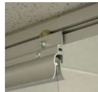
Diagram of a Data Center Curtains containing the airflow in the Cold Aisles
